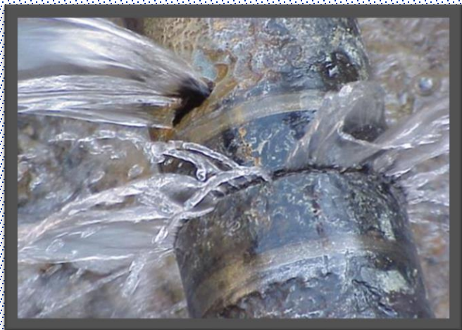
Caused by corrosion and pipe movement
