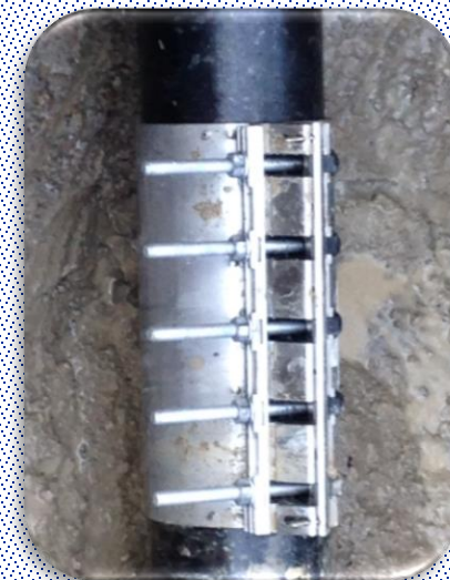
Conventional clamps move stress down the pipes
