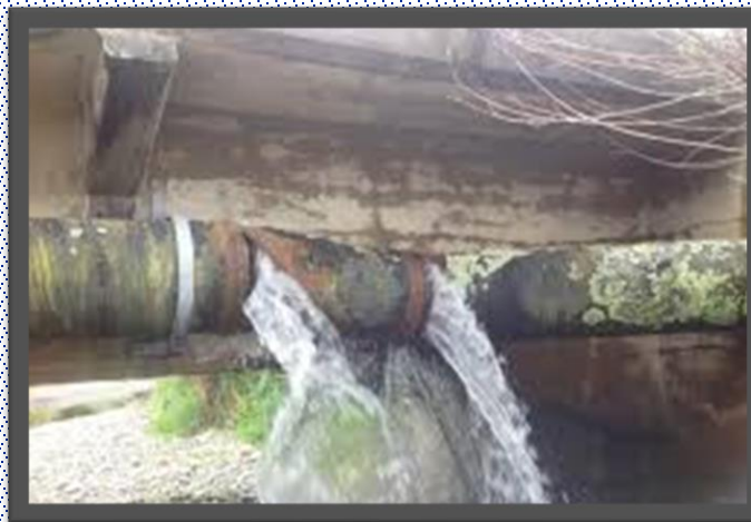
Caused by corrosion and pipe movement
